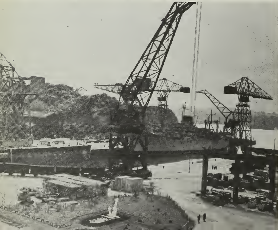
BIRD-LIKE—Cranes in Yokosuka drydock area make repairs on Navy ships.
